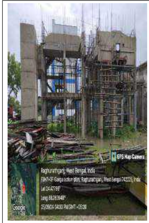
RAGHUNATHGUNJ STP SITE
